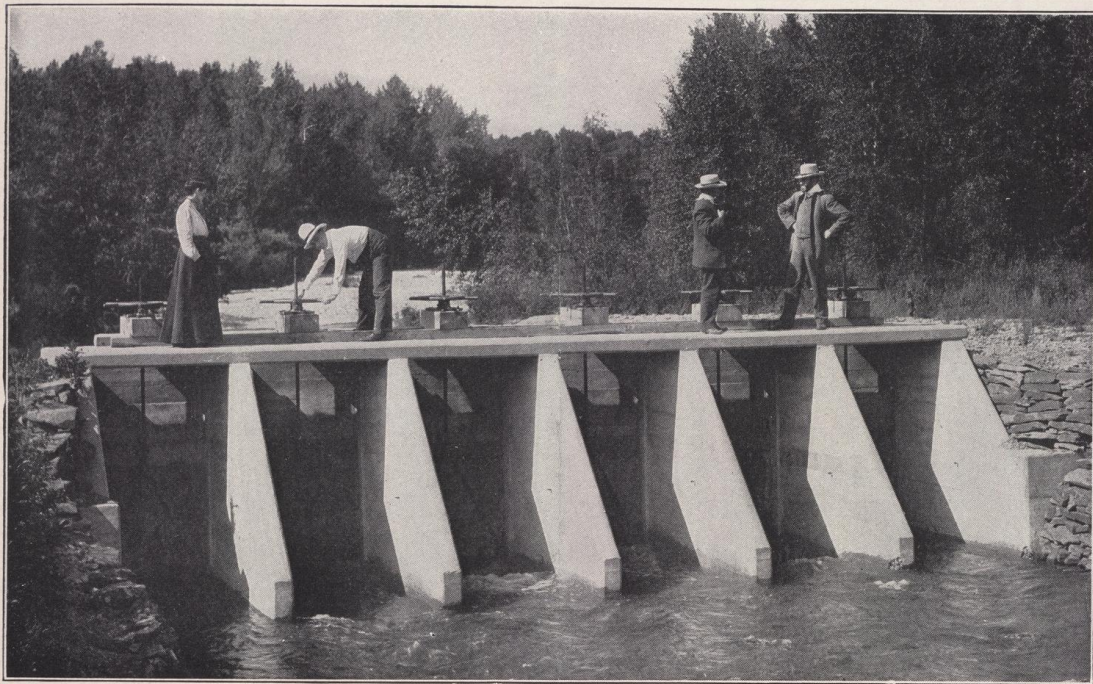
Rear View of Headgate at Intake Canal
