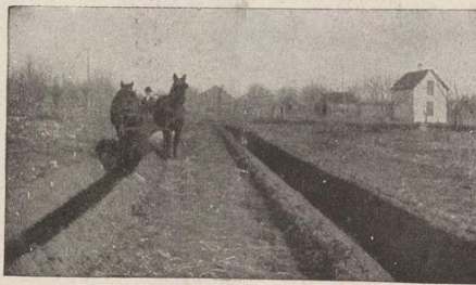
Cutting ditch 20 inches deep, 24 inches wide
