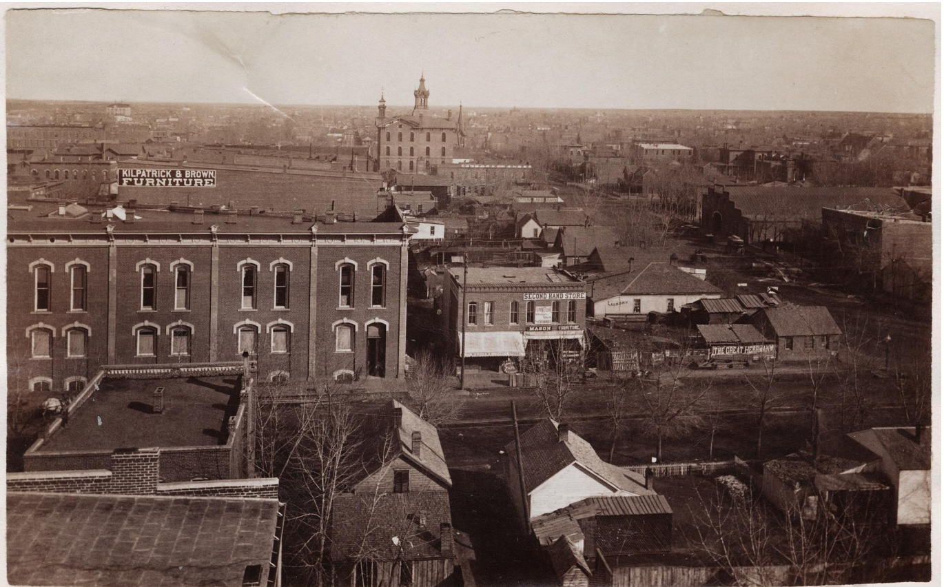
Arapahoe, & 15 th St. (Looking North West.)
