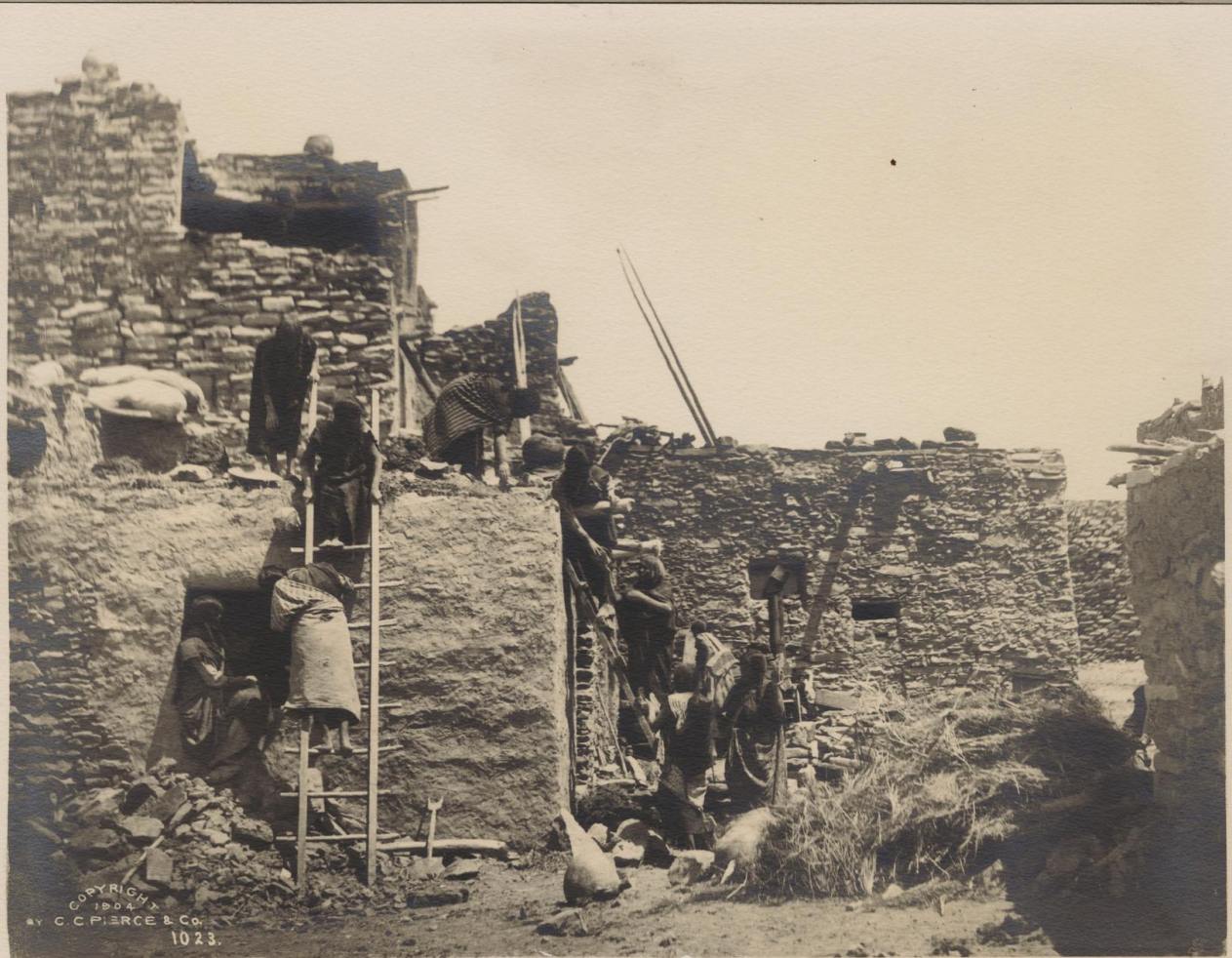
Oraibi women building a house, Hopi Reservation, Arizona.
